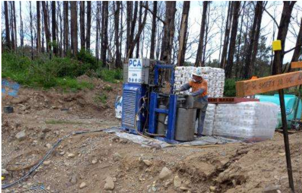
On-site grout mixing station for rock anchors up on banks away from anchors
