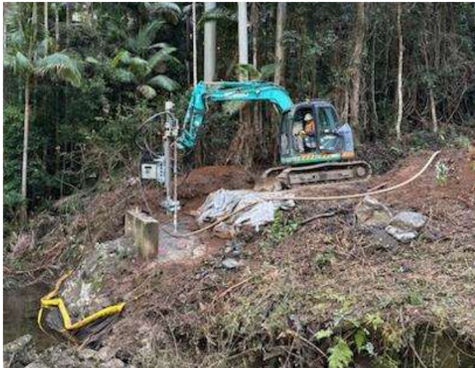
Same smaller excavator (7t) rock anchor rig
