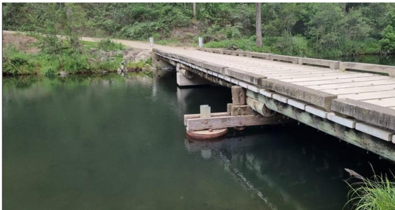
Plate 1.3 Justins Bridge – existing timber structure
