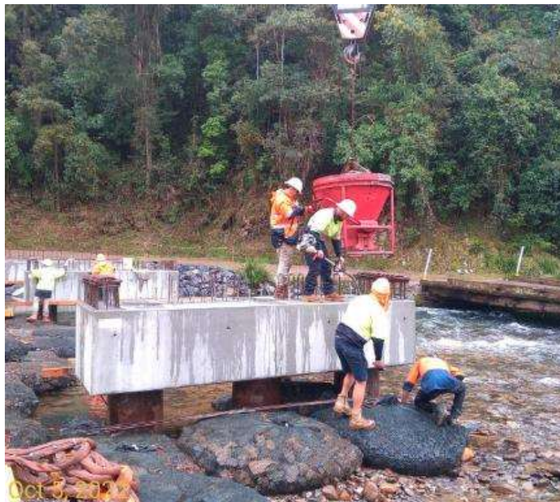
Kibble being used for on-site pours at headstocks near water to control concrete
