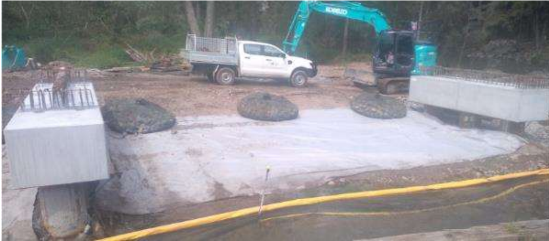
Rock bags used to pin down geofabric with boom adjacent in water
