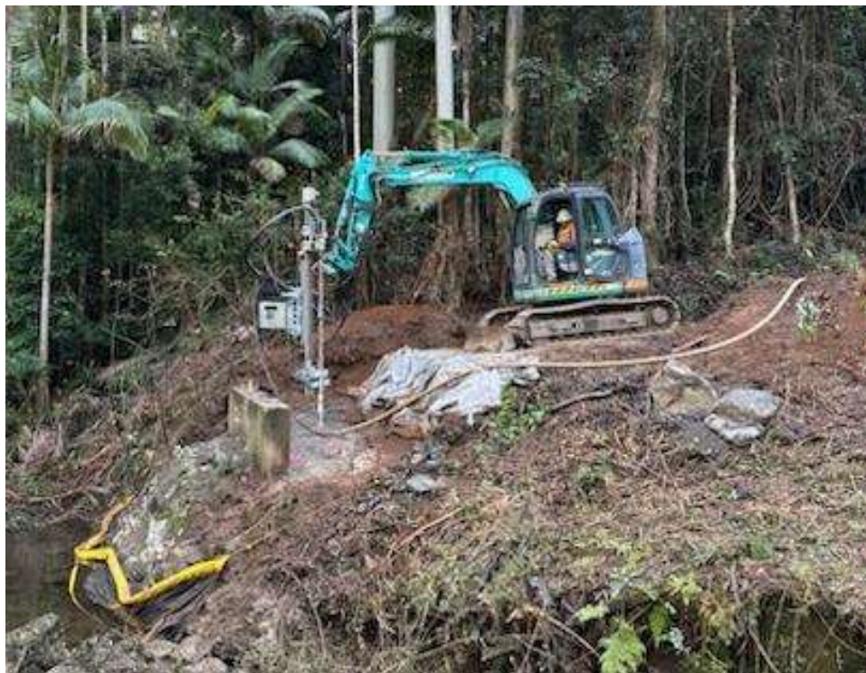
Same smaller excavator (7t) rock anchor rig
