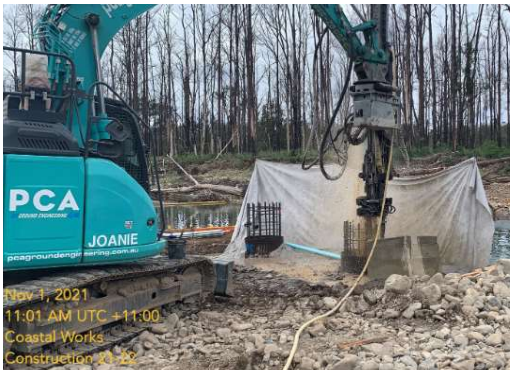
Excavator mounted rock anchor drilling setup (7-12t sized machine) with splatter screens used next to waterway
