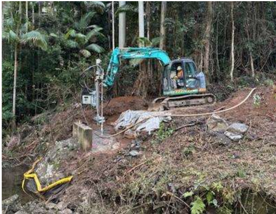
Same smaller excavator (7t) rock anchor rig
