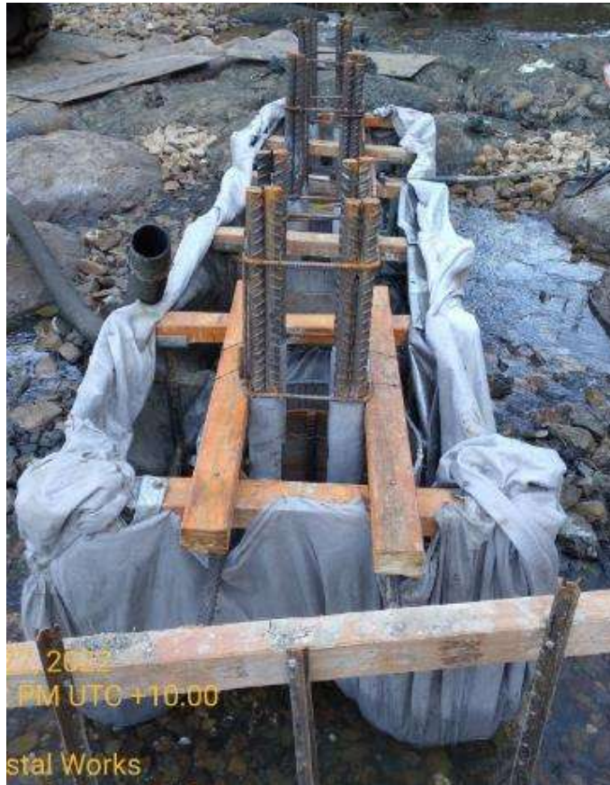
Containment system used for pouring concrete bored piles to prevent concrete overpour entering the waterway
