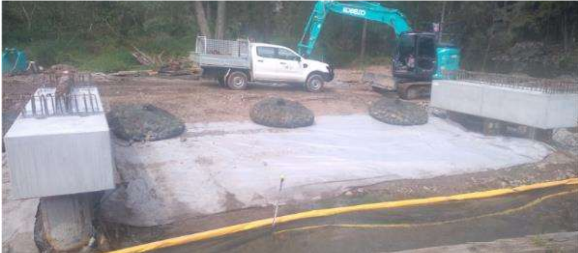
Rock bags used to pin down geofabric with boom adjacent in water
