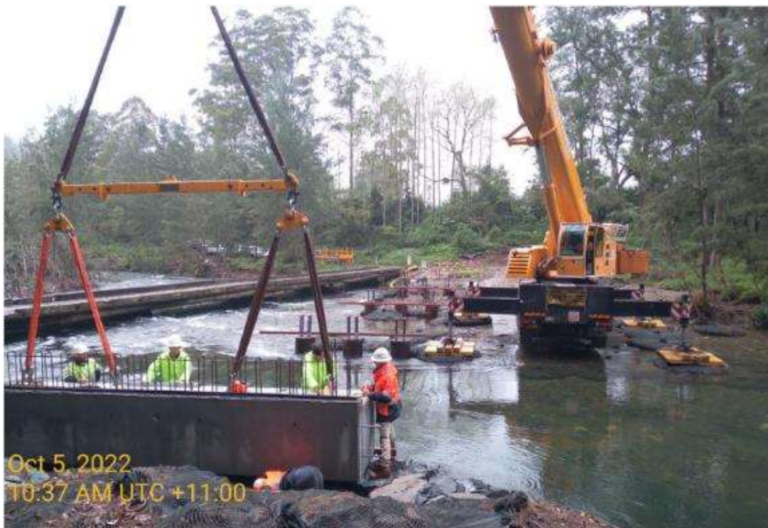
Rock bags used as an access track and crane platform for landing precast components
