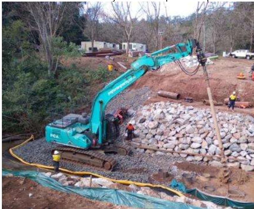
Excavator mounted pendulum pile boring rig with extendable Kelly bar and access ramps –
